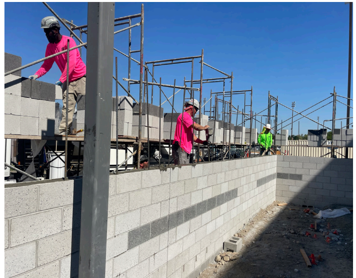
Aden Masonry laying CMU block in the residential inpatient courtyard.
