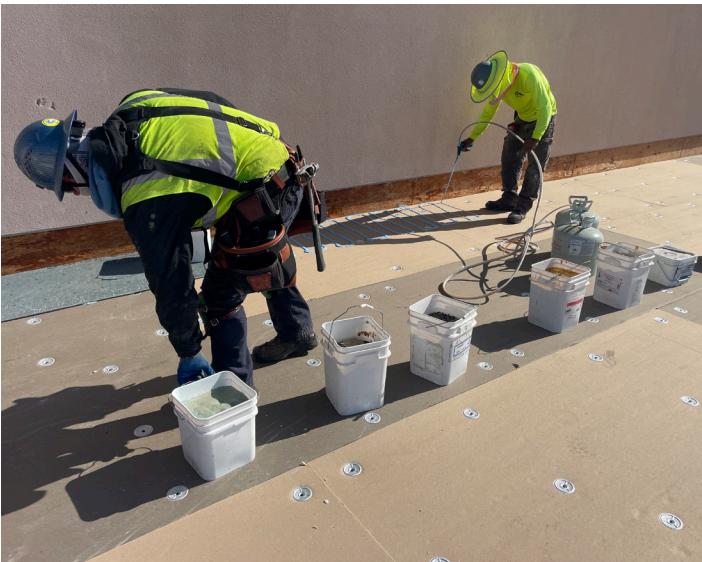
Palmer Roofing installing the roof overlay south of penthouse.
