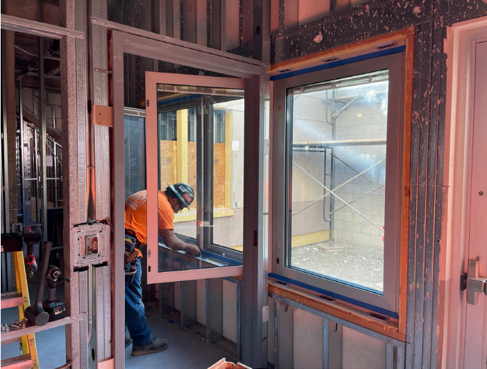
Perfection Glass installing the Wasau windows in 23-hour observation.
